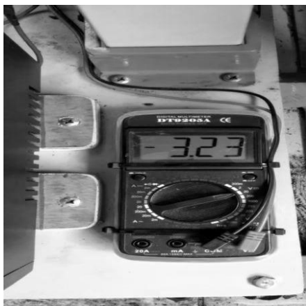
Fig .15. Multimeter voltage output with load (battery)
