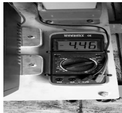
Fig. 16. Multimeter voltage output without Load (Battery)
