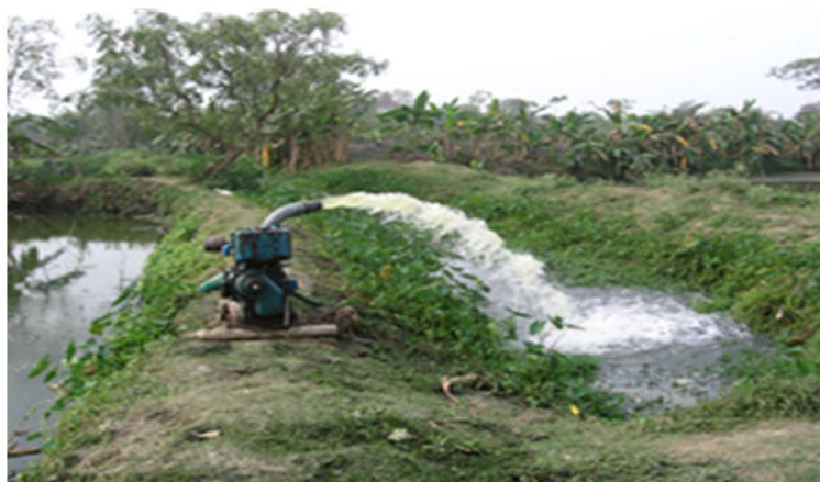
Fig. 5. More recent practice of pumping wastewater from secondary canals to stabilization ponds
