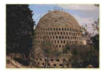
Fig. 1. Sight sud/est of the "bell" of the air well with its 5 line of partly high ventilation
